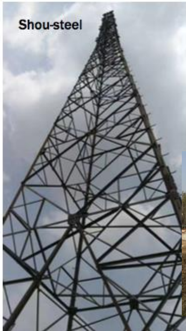
安徽铁塔（首钢）460MPa, 2017, demo tower in Anhui
