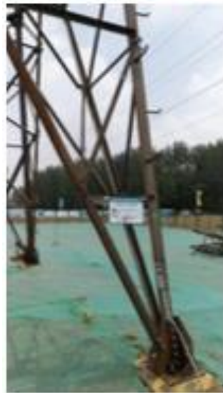
安徽铁塔（首钢）460MPa, 2017, demo tower in Anhui
